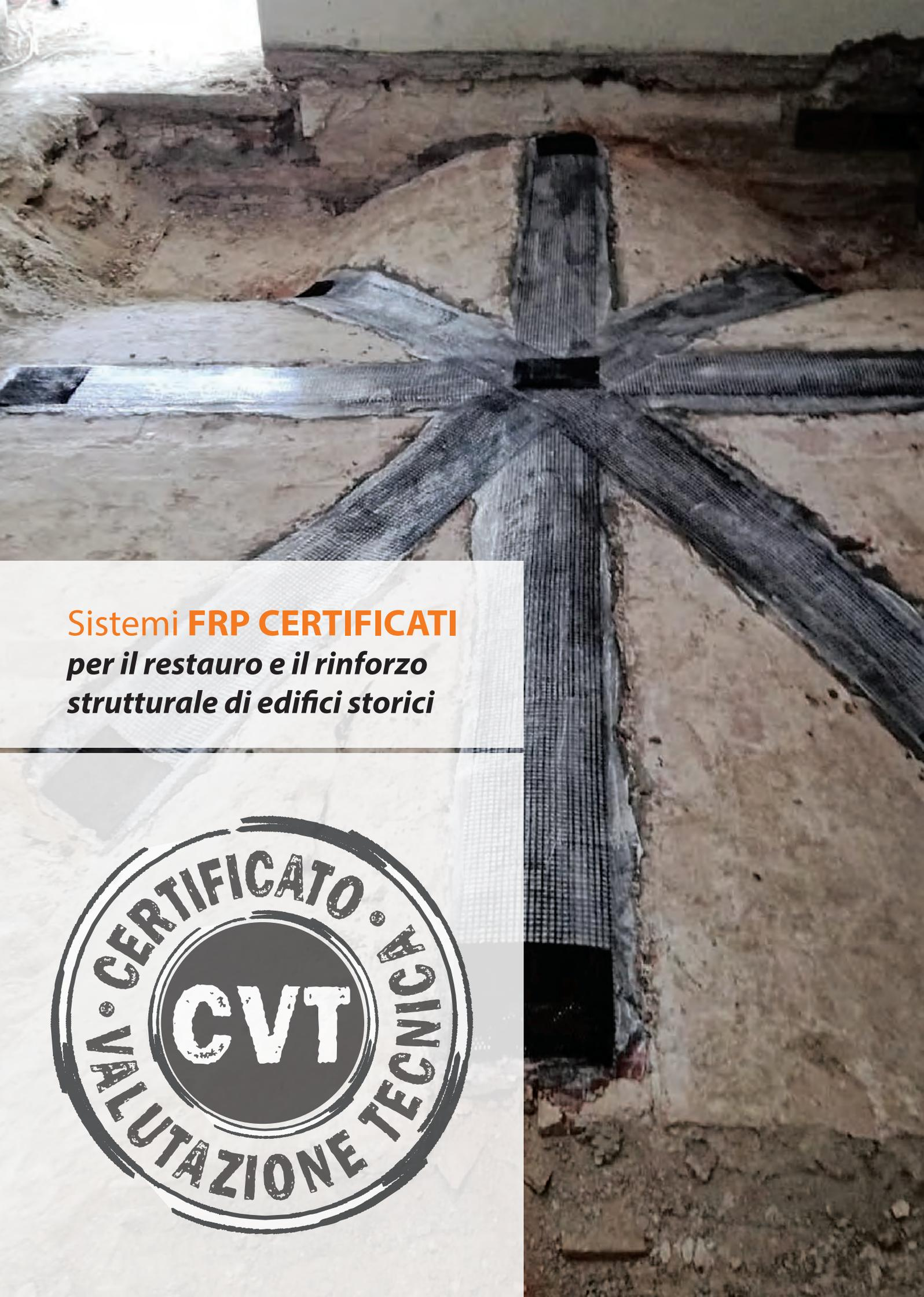
A photograph showing several grey, fibrous FRP strips applied to a concrete surface. The strips are arranged in a star-like pattern, radiating from a central point. The concrete appears to be part of a larger structure, possibly a wall or ceiling, and shows signs of wear and cracking. The lighting is somewhat dim, highlighting the texture of the FRP strips.
